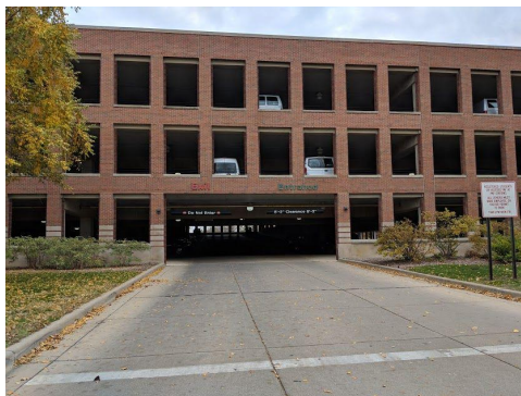
View of entrance to Ramp #5 from Red Cedar Road
